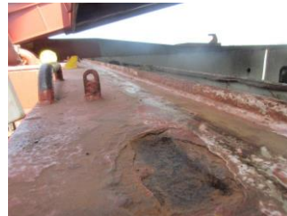
Bearing pad, coaming table side (not reinforced)
