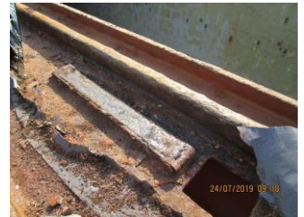
Bearing pad, coaming table side (pad structure)
