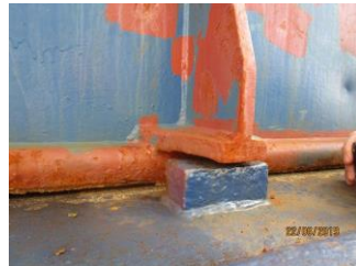
Bearing pad ensemble - not touching
