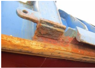
Bearing pad, hatch cover side
