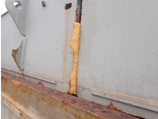
Expansion foam between panels
