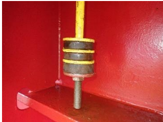
Cleat with additional rubber and steel washers
