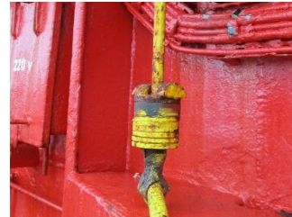
Cleat with additional steel washers
