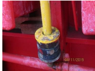
Cleat with additional rubber washers
