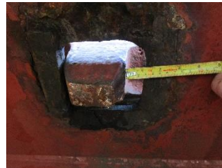
Measuring longitudinal clearance
