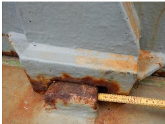
Positioner type with pin on coaming
